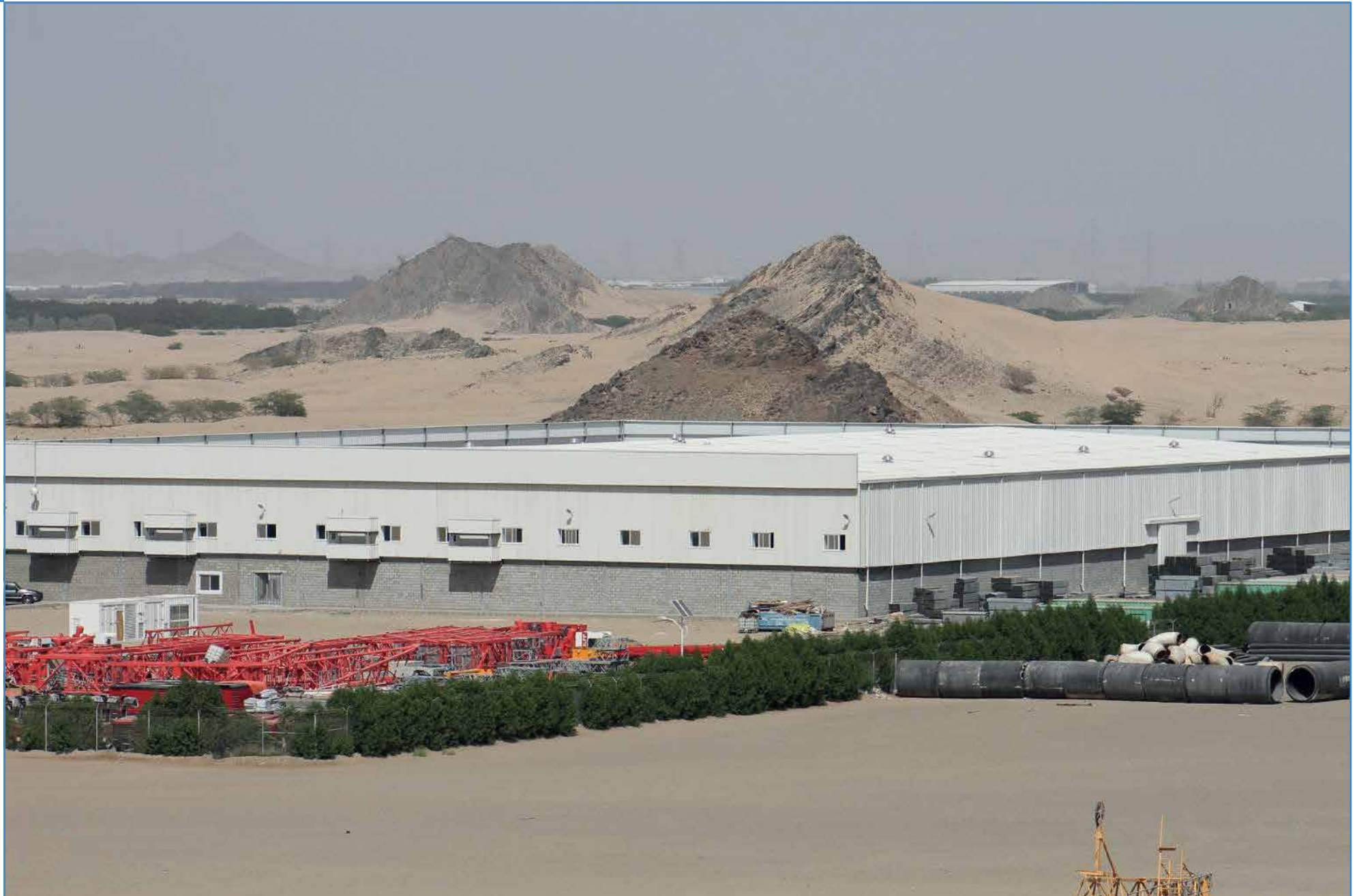
Bahra Warehouse Project / Makkah
