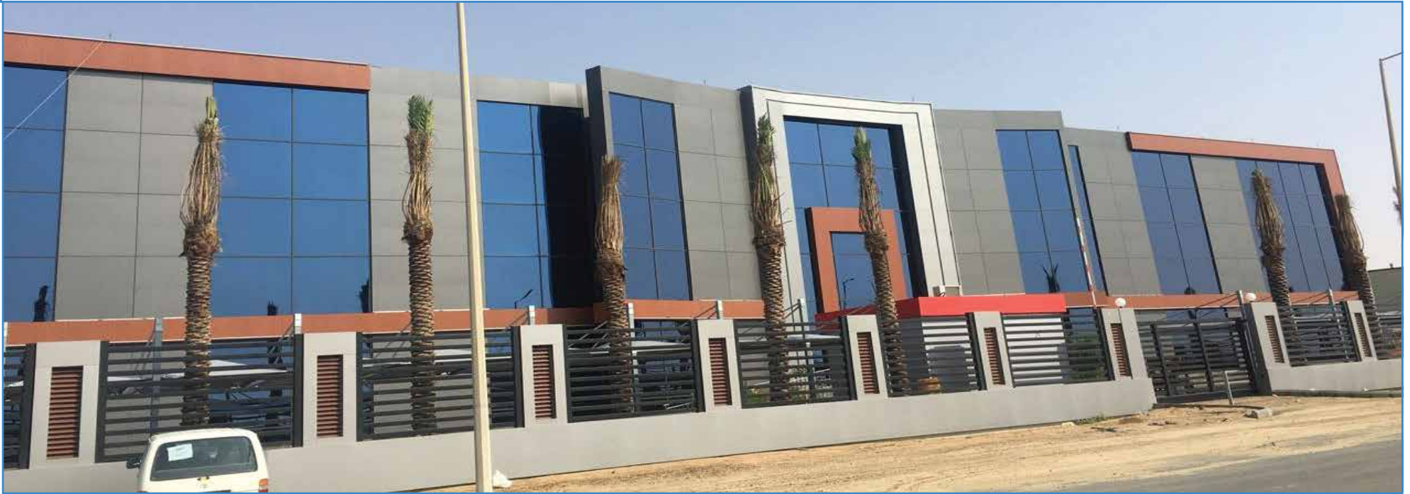
Alesayi Beverage Corp. Factory / Jeddah
